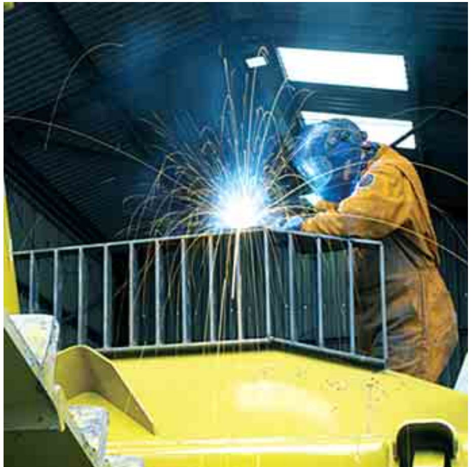
Plant maintenance is undertaken by a team of manufacturer supplied and our own in house fitters.
